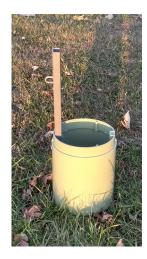
**4.** Push the stake on the bottom half of the cable box into the ground. (see Warning below)
